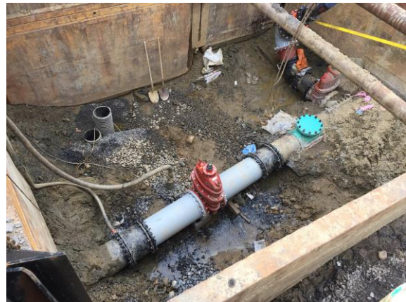
Westtown Way PS New Isolation Valve
